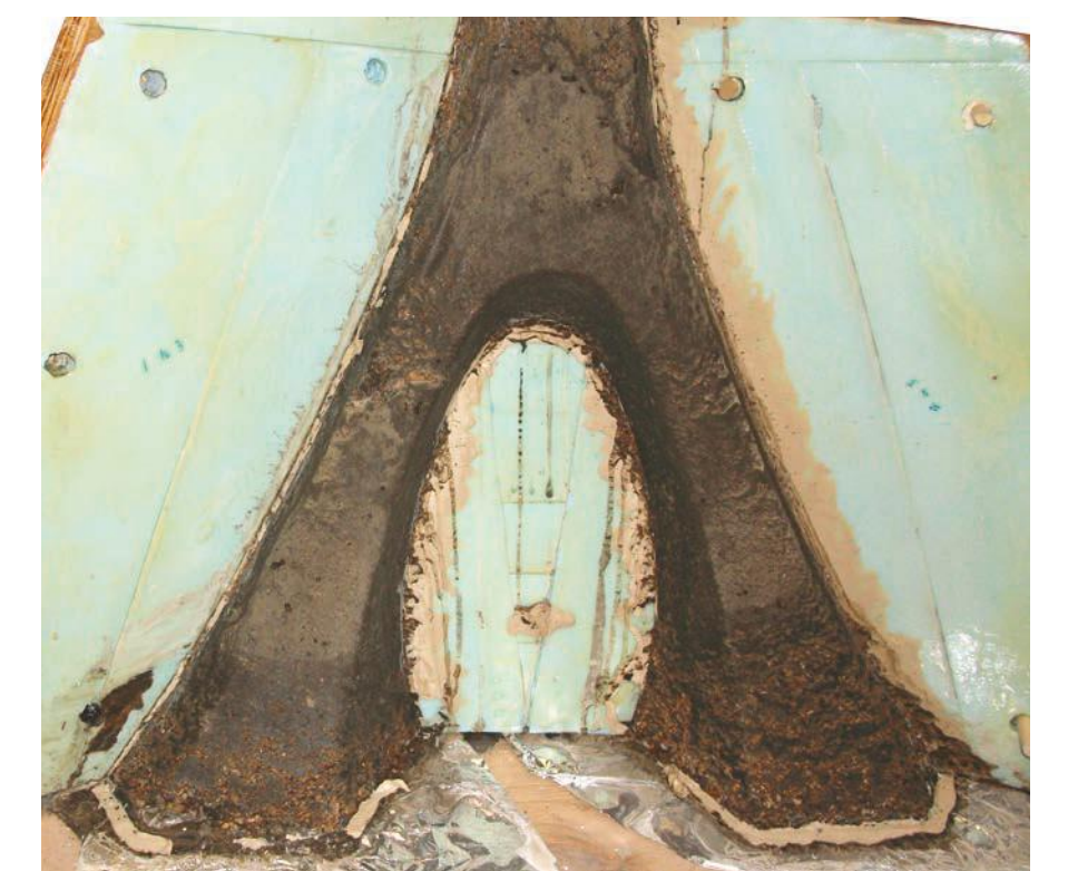
AGGREGATE ACCUMULATION AT BASE
