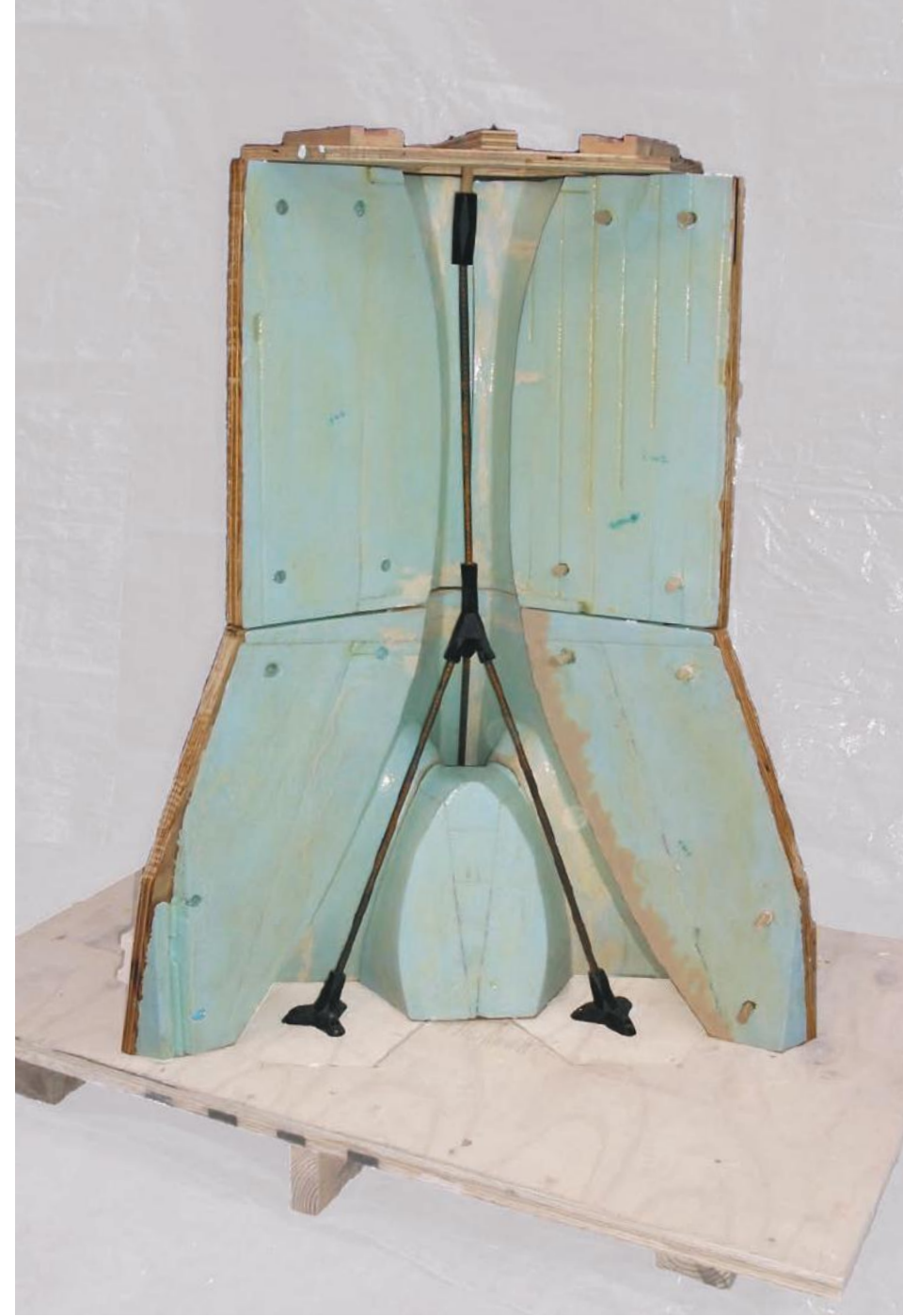
REBAR POSITIONING IN FORMWORK
