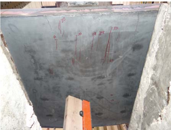
Cracking at Loads
