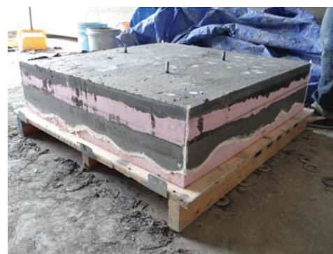
PANEL AFTER FORMWORK PULLED
