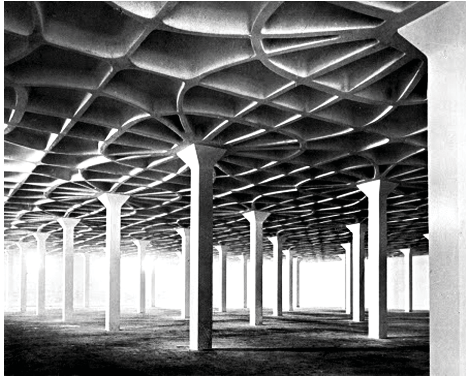
Luigi Nervi Gatti Wool Factory, Rome - Ribs following the isostatic lines of the principal bending moments.
